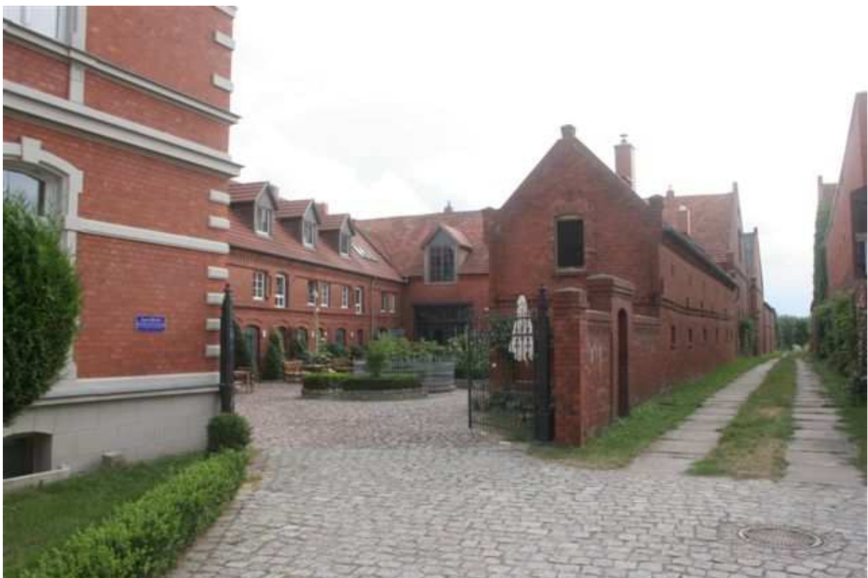
The pension in Garz, installed in a thoroughly renovated Farm house.
