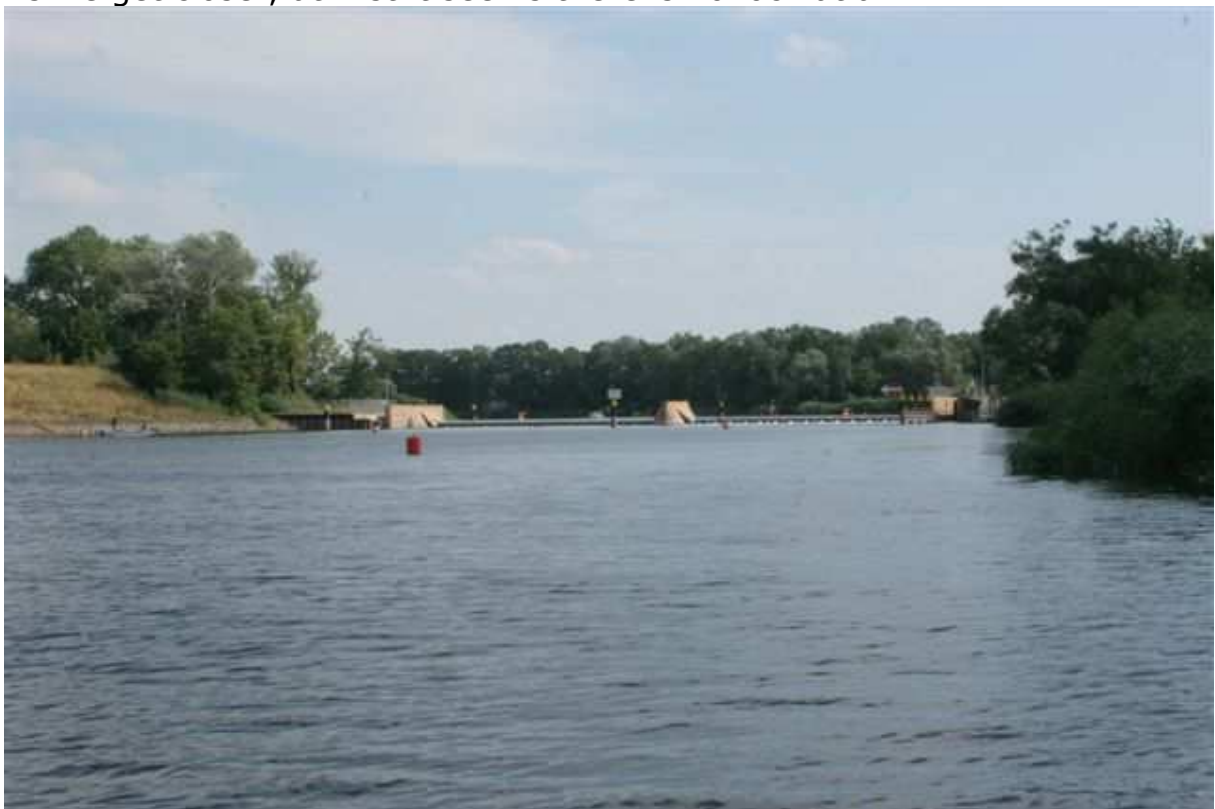
The weir at Bahnitz.
